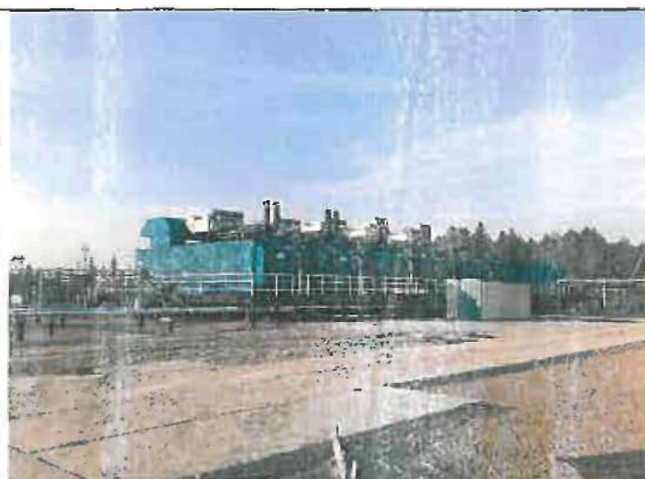
Figure 1. Project Gas Power Plant (GPP).
