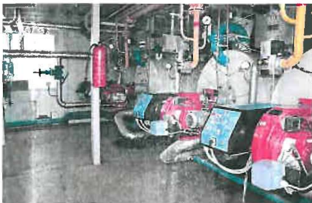
Figure 4. Heating station at Vostochno - Perevalnoye oilfield.
